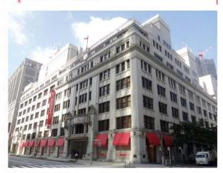
Mitsukoshi Main Store has been extended repeatedly around WWII, based on the original steel-framed reinforced concrete building (7-story, one-basement) completed in 1927. The high-quality design features the exterior that takes the classical Western style, and the interior such as the richly-colored Mitsukoshi Hall and the Art-Deco style hall.
