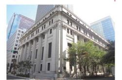
Completed in 1929, Mitsui Main Building opened as the headquarter office building of Mitsui Gomei Kaisha, Mitsui Bank, Mitsui Trust, and Mitsui Mining to name a few. The steel-framed reinforced concrete building (7-story, 2-basement) features the Corinthian order and the Doric order pillars lining up at the soaring interior lobby.
