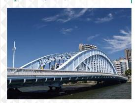
Eitai Bridge, rebuilt as part of the capital's recovery project from the Great Kanto Earthquake, was completed in 1926. At time of construction, it was a steel truss bridge that achieved a high level of technical perfection that achieved the longest span in Japan. The solid rib-arch bridge, characterized by its massive architecture, spans over Sumida River and has a design contrasting Kiyosu Bridge.
