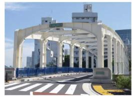
Toyomi Bridge, a bridge built as part of the recovery project from the Great Kanto Earthquake that spans over the mouth of Nihonbashi River, is a through-truss steel Vierendeel bridge built in 1927. Its appearance, which looks like muscular components arranged in a grid-like formation, was designed to balance with the neighboring, massive-looking arch bridge, namely Eitai Bridge. This type of bridge is rare and very few in Japan.
