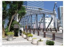
Minami-Takabashi Bridge, a steel truss bridge over Kamejima River, is one of the bridges that were built in 1932 as part of the recovery project of the Great Kanto Earthquake. When the triple-truss Ryogoku Bridge, completed in 1904 was reconstructed, the center span part were relocated and reinforced to create Minami-Takabashi Bridge. It is a valuable bridge diverted from the former Ryogoku Bridge of the Meiji era and still being used to this
