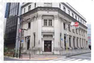
Completed in 1932, Hario Glass Building is a reinforced concrete building that used to be a bank branch office (Kawasaki Savings Bank and Joyo Bank). The exterior design takes the classical Western style, surrounded by fluted Corinthian orders, and the splayed northwestern corner features both Ionian and Doric styles.
