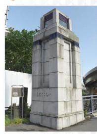
The newel post of Ichikokubashi Bridge that marked the separation point of the Outer Moat and Nihonbashi River. It is the newel post from 1922 when the bridge was renovated to reinforced concrete arch bridge, part of which survived the Great Kanto Earthquake one year later. It conveys to this day the remnant of the robust old Ichikokubashi Bridge that used granite for the exterior walls.
